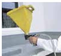
10 ... soffiare Triflex Micro Chips.
